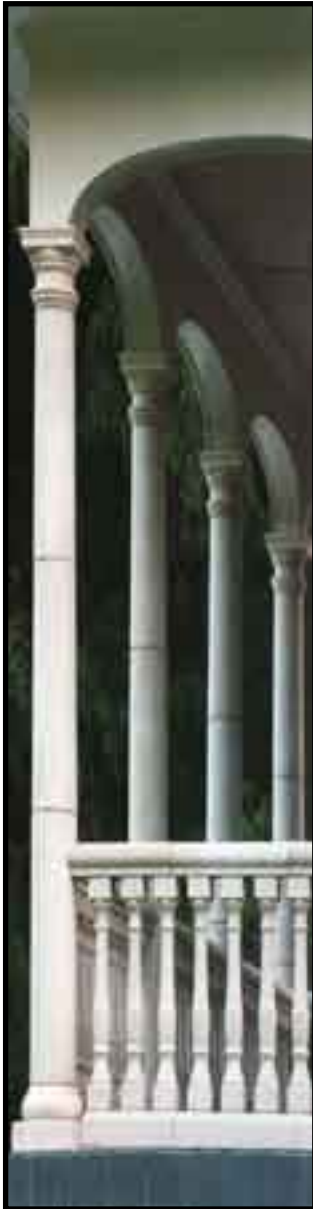
Above is a Tuscan tapered hollow column, installed.
