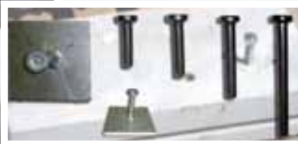
Weld plate imbed and nelson bolts. Used commercially in most cases.
