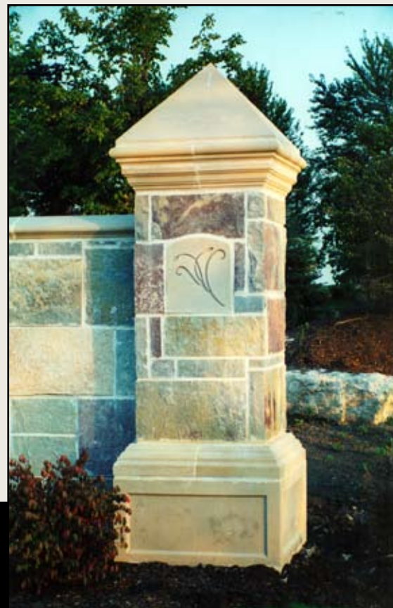
Decorative panel set in landscape pier, with cast stone pier cap and base
