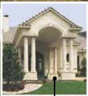
EntryPsrticoEyebrowColumnDouble-Sided Aegean Palace Unit ID 13859
