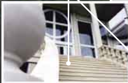
Stair Helical Jefferson1A Connelly1 Cove1 UnitID 14196
