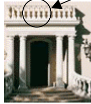
Top Right: Setting line used in a Balustrade System
