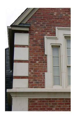
Quoins - Cast stone block used to make up a corner of a wall.
