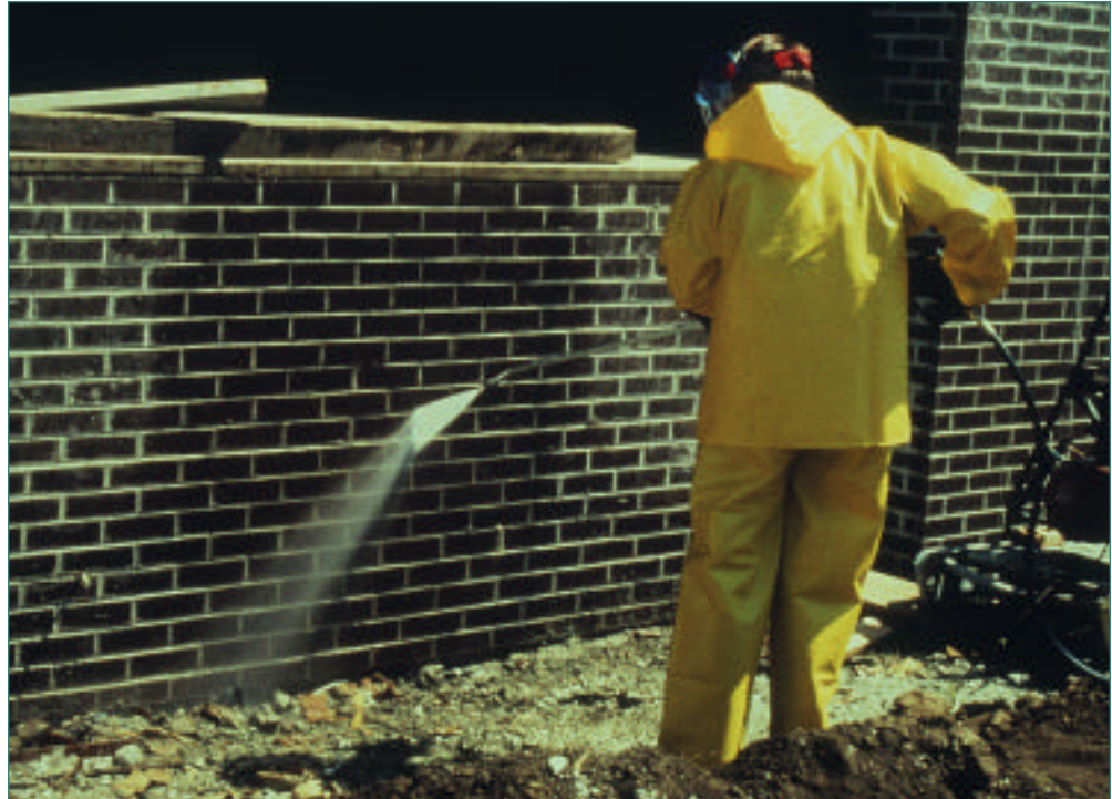
Figure 5. If efflorescence must be removed chemically, walls should be thoroughly rinsed to remove all traces of the cleaner. (70029)
