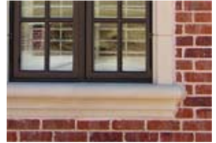
EXAMPLE PHOTO OF SILLS
