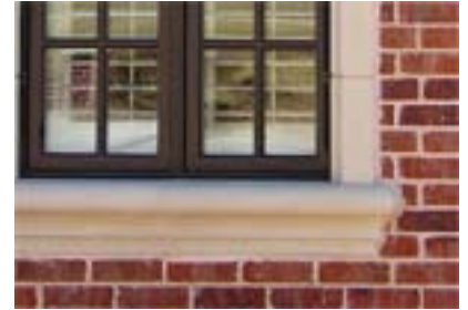
EXAMPLE PHOTO OF SILLS
