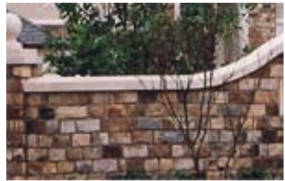
EXAMPLE PHOTO OF WALL CAP
