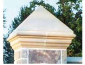
EXAMPLE PHOTO OF PIER CAP
