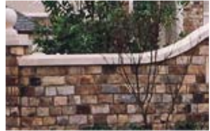
EXAMPLE PHOTO OF WALL CAP
