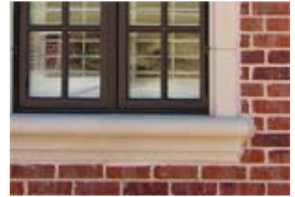
EXAMPLE PHOTO OF SILLS
