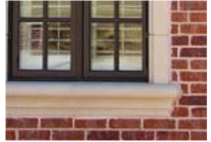
EXAMPLE PHOTO OF SILLS
