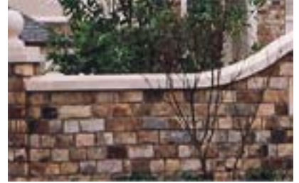
EXAMPLE PHOTO OF WALL CAP
