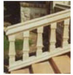
EXAMPLE PHOTO OF BALUSTRADE
