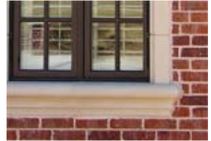
EXAMPLE PHOTO OF SILLS
