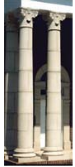
EXAMPLE PHOTO OF COLUMN
