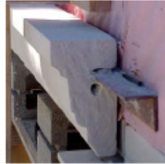
Steel angle lintel inserted into the back of the stone.
