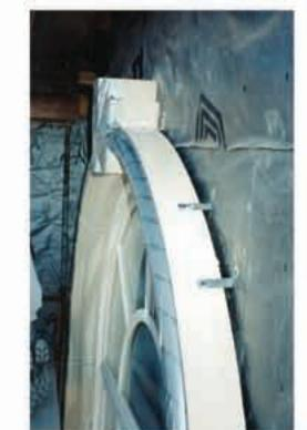
Above, securing a circletop surround using strap anchors and tapcon screws.
