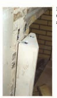
Left, a fireplace leg using strap anchors and tapcon screws.
