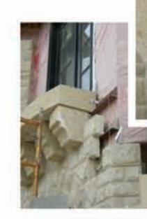
Left and above, an excellent example of clip anchors and steel lintels used in a surround installation.
