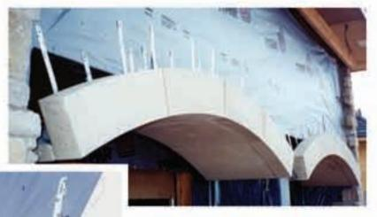
Left and above, securing a circletop surround with soffit using strap anchors and tapcon screws.
