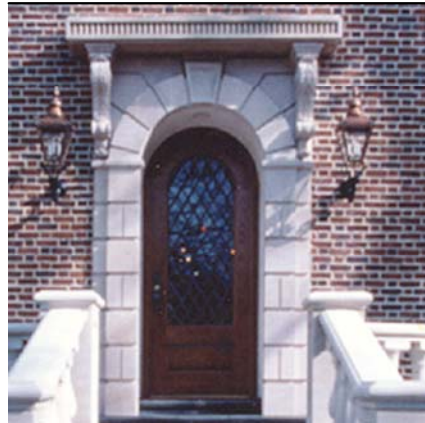
This "Recess" Keystone was designed to fit the pattern of the entry.
