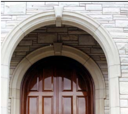
Note the wider Chamfer Keystone on the Circle Top Door surround in comparison to the one on the front of the building
