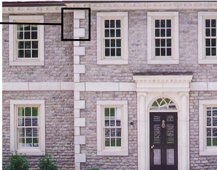
Alternating Staggering Corner - Flatface Note how the quoins compliment the flatface banding.
