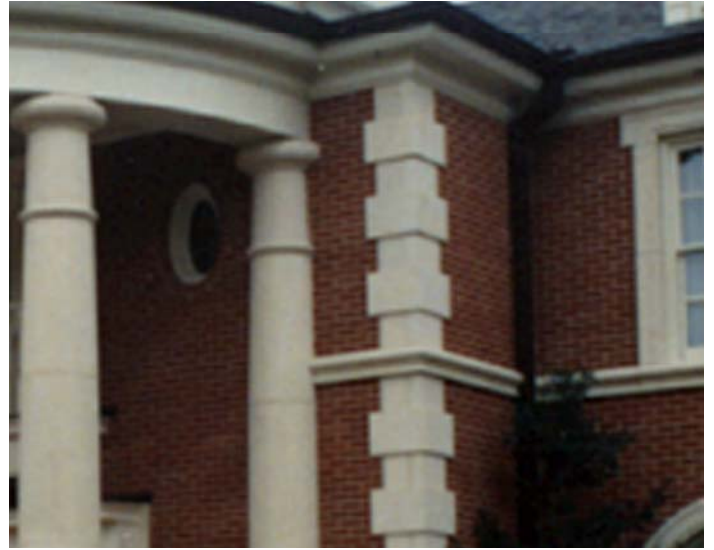
Alternating Staggering Corner - Flatface Note alternating stone depth.
