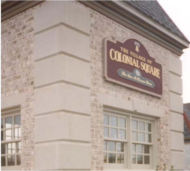
Stacked Corner - Chamfer
