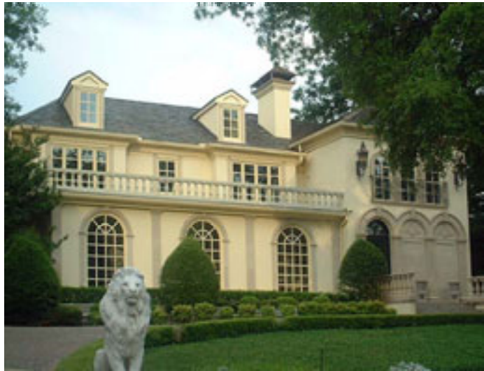
Note the Pilasters Between the Windows and on the Entry of the House
