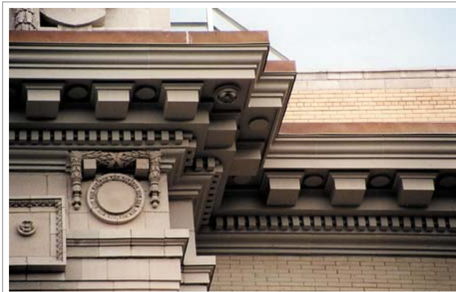
Architectural Fiberglass Corp. replicated the cornices on this New York City apartment building using fiberglass.
