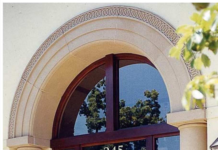
Architectural Facades Unlimited fabricated this precast arched entry surround for the Lytton Building in Palo Alto, CA.
