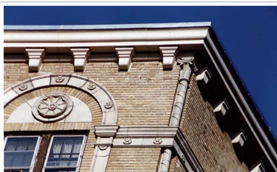
Architectural Fiberglass Corp. fabricated the dentils and brackets for the Yonkers City Hall building in Yonkers, NY.
