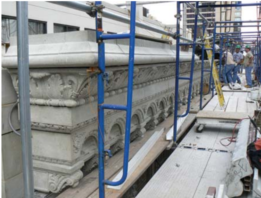
For this project, Towne House Restorations replaced a terra-cotta cornice with GFRC.
