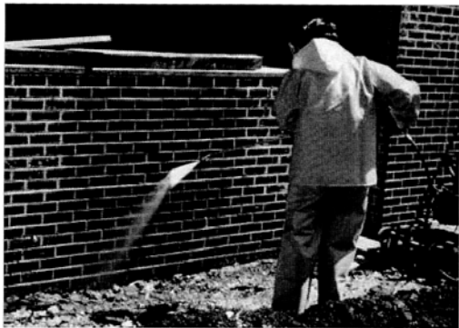
Figure 5. If efflorescence must be removed chemically, walls should be thoroughly rinsed to remove all traces of the cleaner. (70028)
