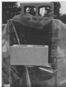
Figure 4. The top of masonry walls should be protected with a tarp whenever rain or snow is expected. It is good practice to cover work at the end of each day to help keep excessive water out and aid curing. (70028)
