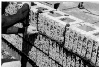
Figure 2. Tooling joints compacts the mortar and creates a weather-tight bond. This minimizes water entry into the wall, which reduces the potential for efflorescence. (70027)
