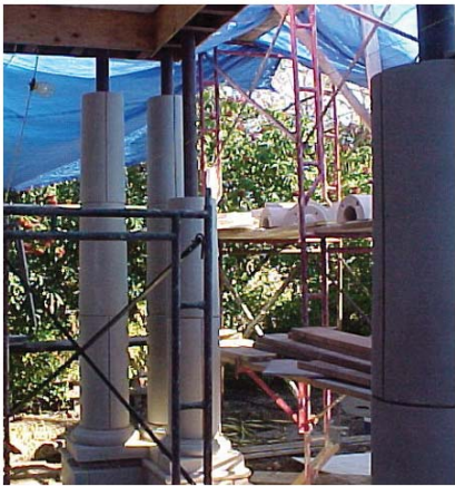
Above, Tuscan Tapered Hollow Smooth Columns during installation.
