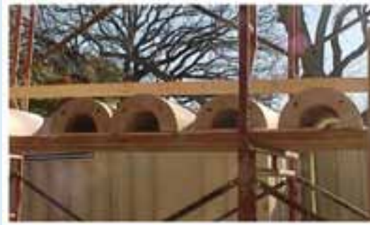
Above, Tapered Hollow Smooth column shafts awaiting installation, note the pre-drilled pin holes.
