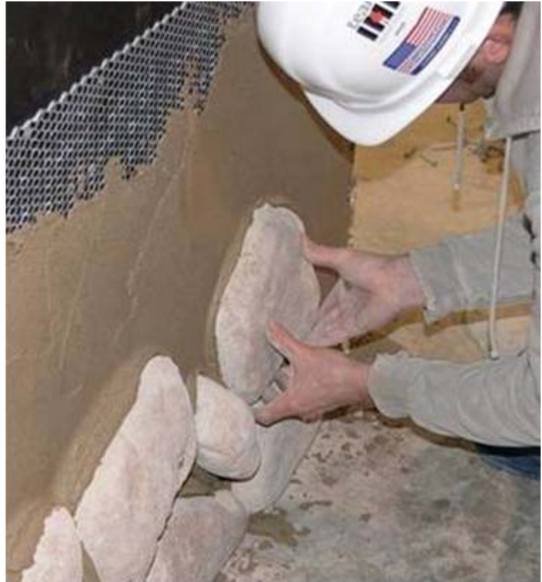
Photo provided courtesy of International Masonry Institute
