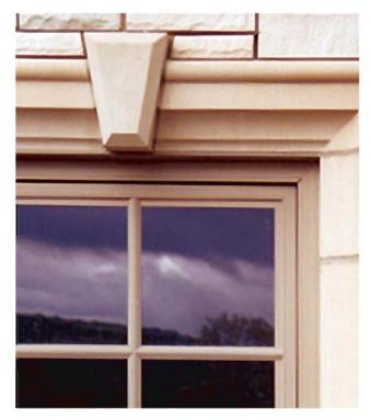
**Keystones** - Originally, the final supporting unit at the center of an arch. It is generally wedge shaped.
