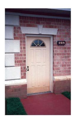
Jack Arches - are structural elements in masonry construction that provides support at openings in the masonry
