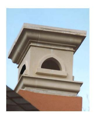
Chimney Caps - a raised cover for the top of a chimney, usually in the form of a slab or cornice.
