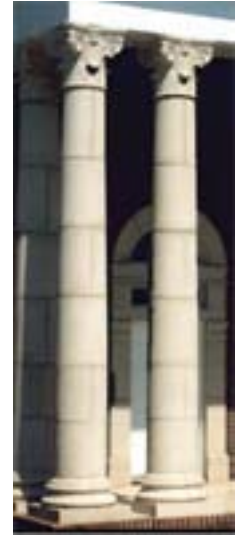
EXAMPLE PHOTO OF COLUMN
