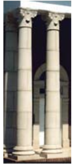
EXAMPLE PHOTO OF COLUMN
