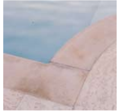
EXAMPLE PHOTO OF POOL COPING
