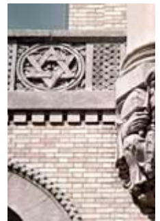
Sculptural ornament in cast stone. Repeating decorative banding course paneled with natural stone. Photo: Richard Pieper.
