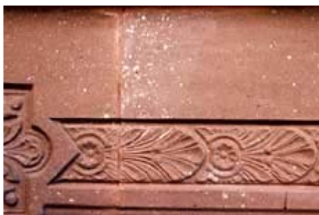
Unlike natural stone, cast stone generally may not be tooled in place to reduce lippage of uneven surfaces at joints. Tooling often exposes coarse aggregate from below the surface. Photo: Richard Pieper.
