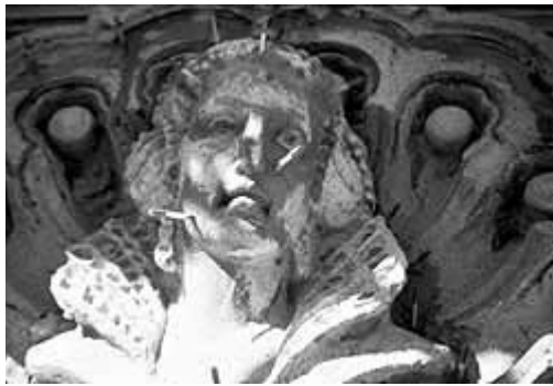
A delaminated layer of ornamental cast stone on the Orpheum Theater, San Francisco, California (1925), was successfully re-attached using epoxy. The multiple delivery ports for the epoxy are removed after treatment and the holes patched. Photo: David P. Wessell.
