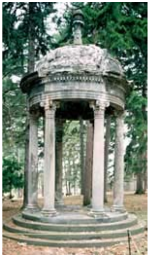
Scaling of cast stone units signals problems with the cementing mix and method of manufacture. Serious deterioration of cast stone, such as this, warrants replacement. Photos: Richard Pieper.
