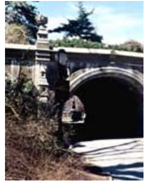
Constructed in 1868 of Belton Stone, the Cleft Ridge Span in New York City is one of the earliest extant cast stone structures in the United States. Photo: Richard Pieper.
