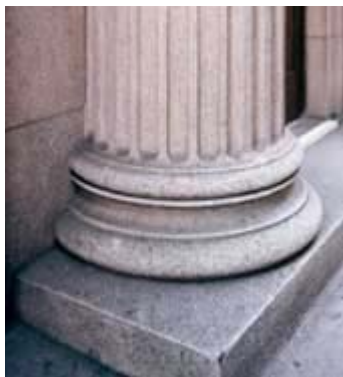
For this column, the appearance of a "pink granite" was simulated by using a pinkish matrix with white and black aggregate. Erosion of a tinted matrix results in a significant lightening of the cast stone surface. Photo: Richard Pieper.
