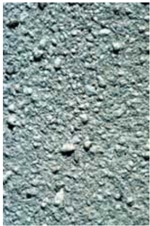
Sandblasting and wet grit blasting can seriously erode the surface and should not be used to clean cast stone surfaces. Photo: Richard Pieper.
