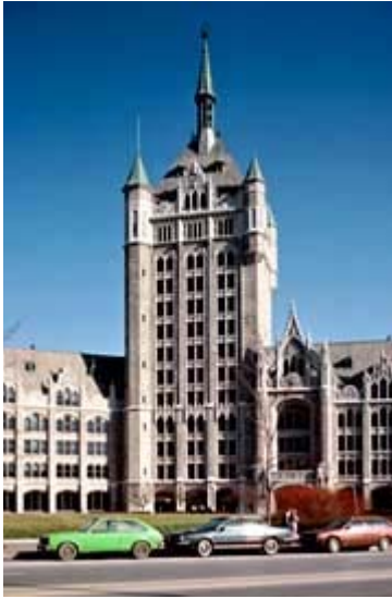
The prominent Delaware and Hudson Building, Albany, New York, (1916) made extensive use of cast stone as trim combined with a random ashlar facing of natural granite. Photo: Richard Pieper.
