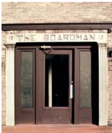
Cast stone was commonly used for molded trim in conjunction with brick or natural stone. This brick building in Rochester, New York, uses cast stone for the entry surround, and natural stone for unornamented windows sills, thresholds, and water table units. Photo: Richard Pieper.
