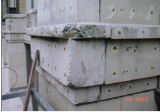
Figure 3 : Surface damage
