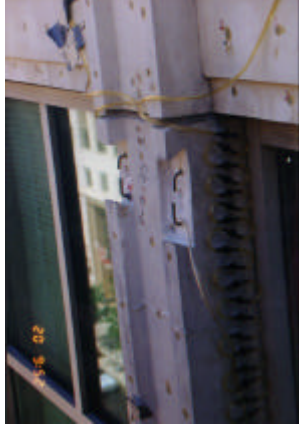
Figure 9 : Epoxy injection, pin installation, and patch preparation
