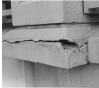
Figure 4 : Cracking at bollard base
