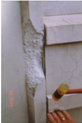
Figure 5: Cracking and spalling of old patches
