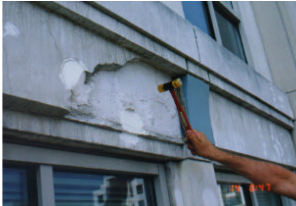
Figure 6 : Delamination of the cast stone at lift line
