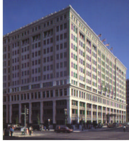
Figure 2 : The current façade
