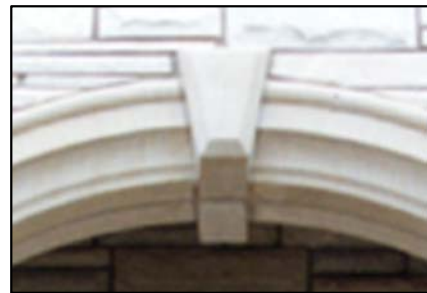
Fitted Keystone after cutting
