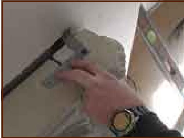
**For security, the stones can be tied together as well as to the wall.**
