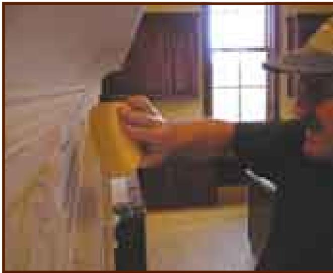
**As the final step, the face of the fireplace is sponged with clean water to remove any grout haze or dirt.**
