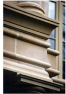
Bandings can be indexed on the "Z" axis (in and out) to create all kinds of designs doing nothing more than stacking profiles. Illustrated is one example of indexing the profiles from the setting line. Indexing is done from the setting line symbol SL (logo) is used in this case to establish the face of the wall. Once the setting line is established all other profiles are aligned + or - the setting line.
