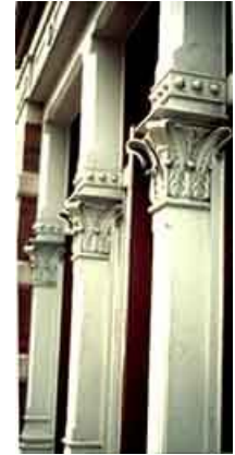
Cast aluminum has been used as a replacement material for cast iron. Photo: NPS files.
