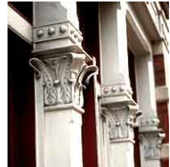
Cast aluminum used as a replacement for cast iron. Photo: NPS files.
