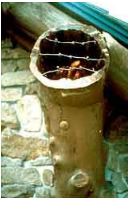
The core of a deteriorated wood outrigger was first drilled out. Photos (left and right): Courtesy, Harrison Goodall.
