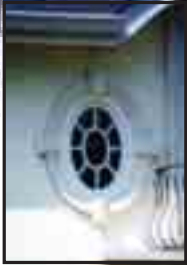
SurroundWindow EllipticalTop Keystone Jamison2A Chamfer UnitID 14746
