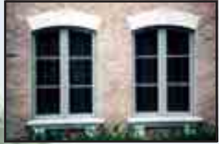
SurroundWindow Eyebrow BracketKeystoneSill Flatface Marsanne1 UnitID 484
