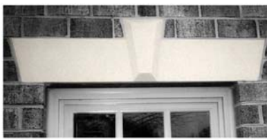
This example shows the very popular Chamfer Keystone in a Jackarch
