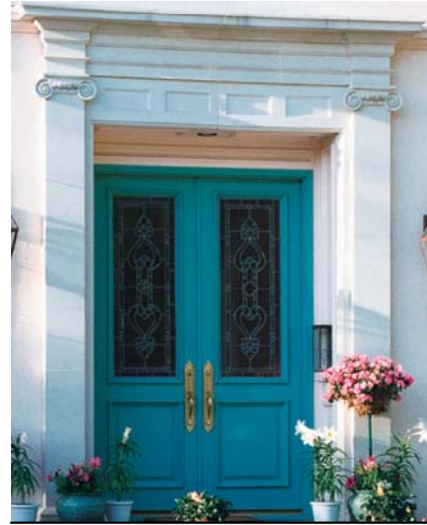
This entry was created with a Lintel, some panels and simple but elegant Pilasters
