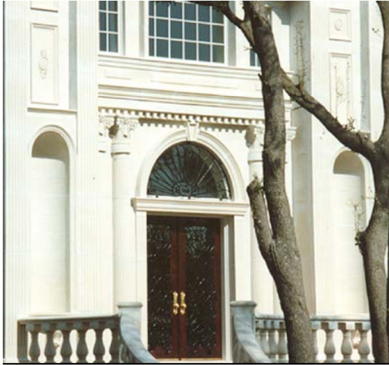
Pilasters of various shapes and sizes can be combined to create an impressive look.
