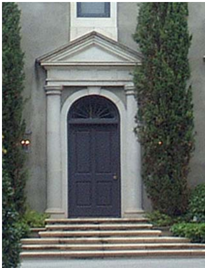
Pilasters and a lintel were used to transform this ordinary door into a great Entry
