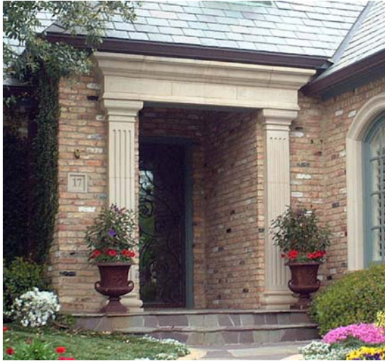
A beautiful example of how an entry can be constructed using a Lintel and a pair of Ariel Flute Pilasters
