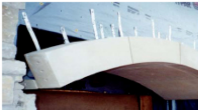
Suspending the stone with straps.
